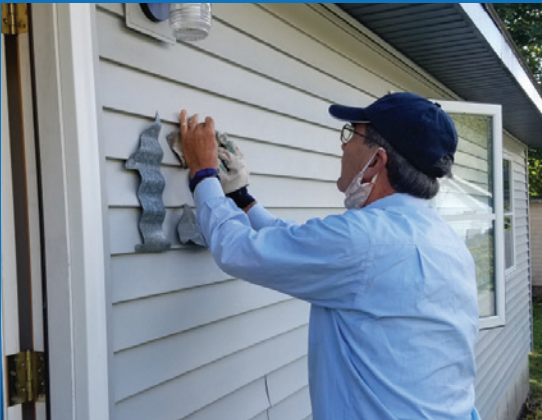
Ted helping put the finishing touches on a 2021 HOAP house.
