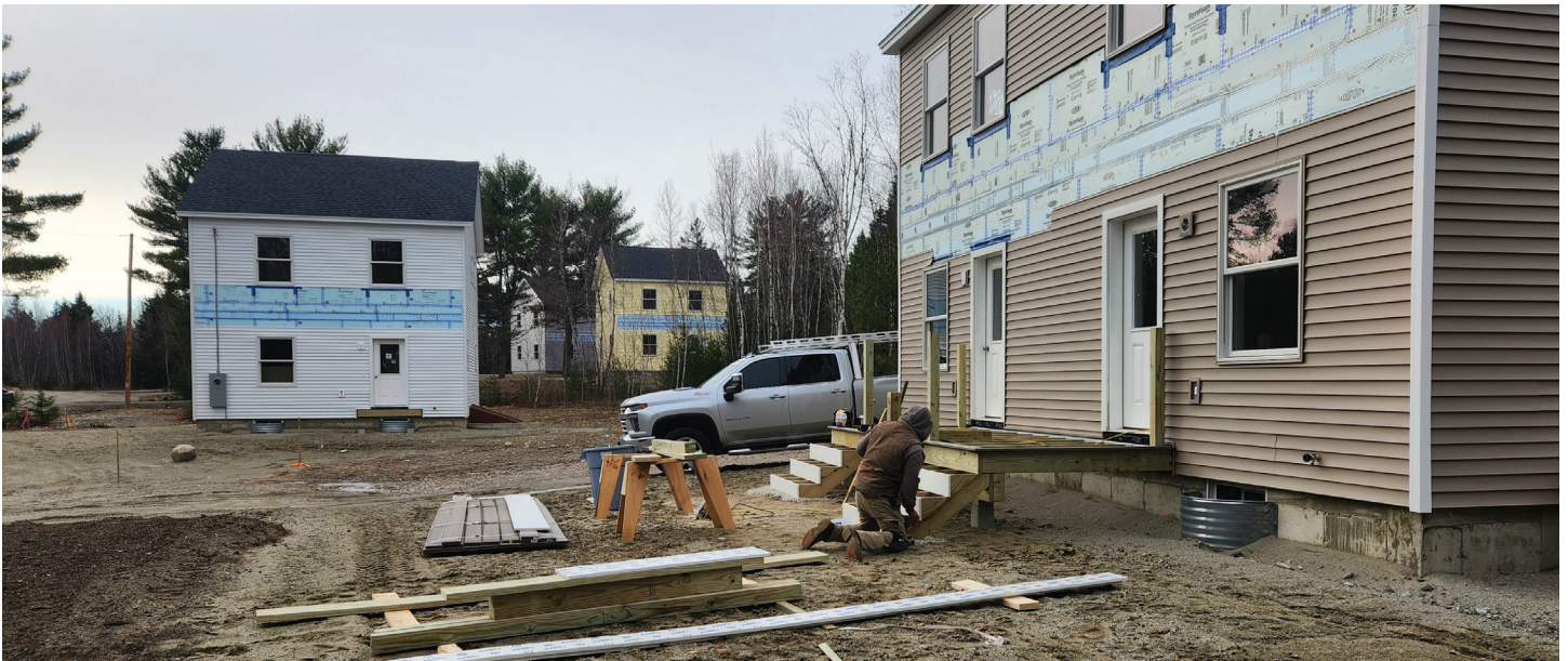
Work continues on a Jones Marsh duplex.
