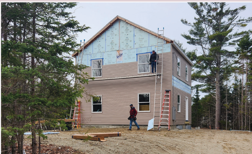
Siding goes up on a Jones Marsh home.
