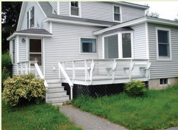
Bar Harbor home under affordability covenants, protected through a partnership with Maine Coast Heritage Trust. IHT photo.
